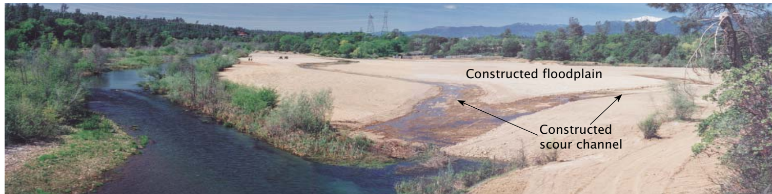
Panorama of Restoration Grove after construction was completed. The scour channel is saturated by groundwater soon after design completion.
